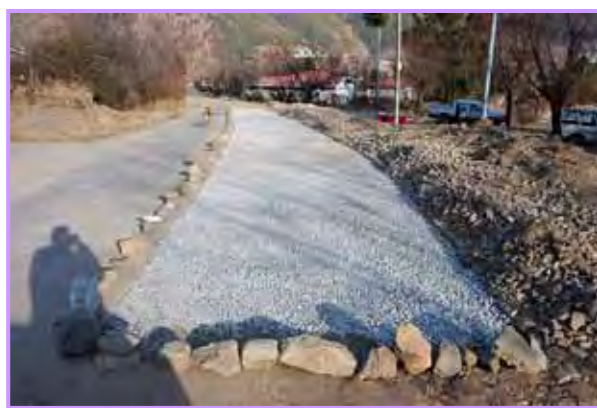
[Photo-24: Road conditions after compacting 12m crushed stone]
