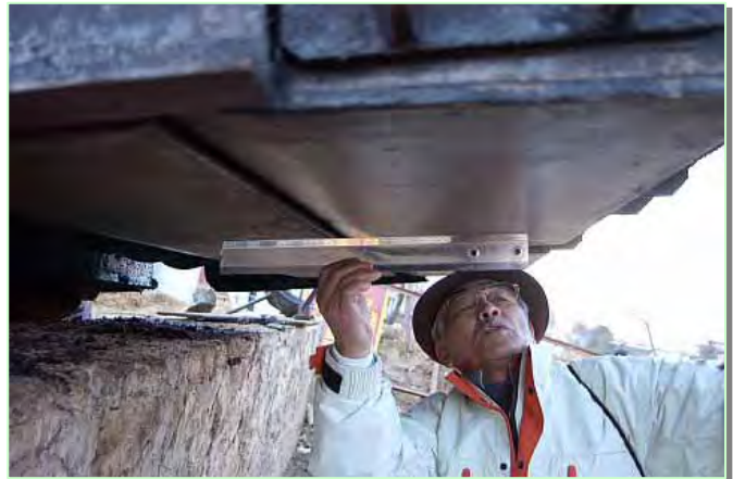
[Photo-10: Inspection of paving machinery]
