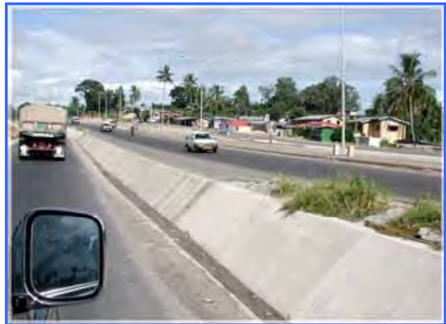
[Photo-45: Road in East Africa constructed with the assistance of Scandinavian government]
