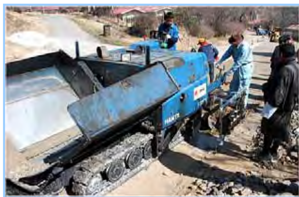
[Photo-26: Field exercise of compacting and shaping with finisher]
