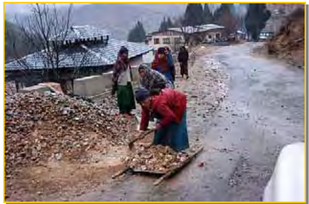
【Photo-4: Road maintenance work at national road】
