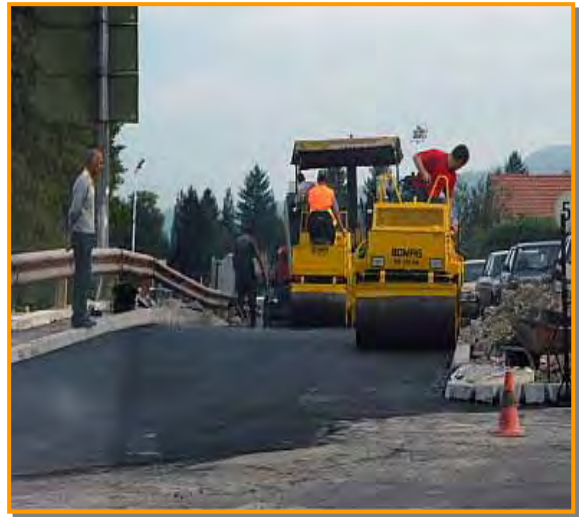
[Photo-37: Compacting with appropriate machinery in Europe]
