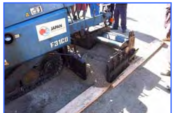
[Photo-18: Adequately filled subbase course material]
