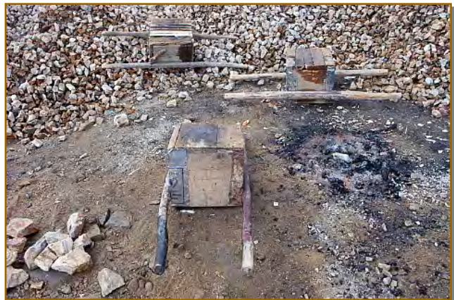
[Photo-13: 1 cft inlet for paving material]
