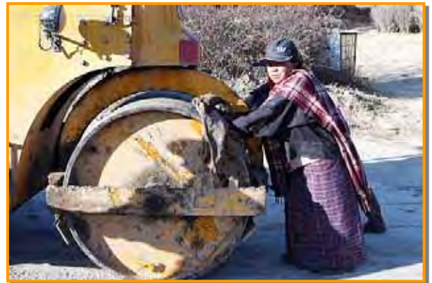
[Photo-28: Compacting after dispersion of emulsion and sand]
