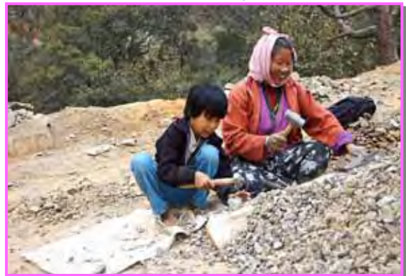
[Photo-39: Stone breaker on site]
