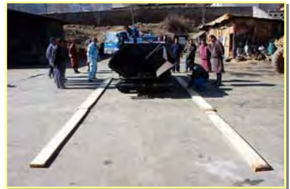
[Photo-17: Setting wooden form for shaping]
