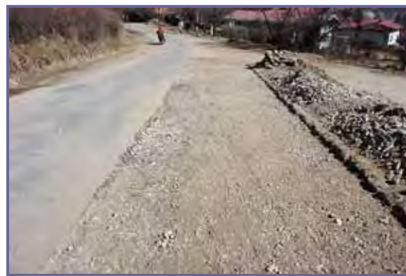
[Photo-23: Road conditions after removal of 30 50mm crushed stone]
