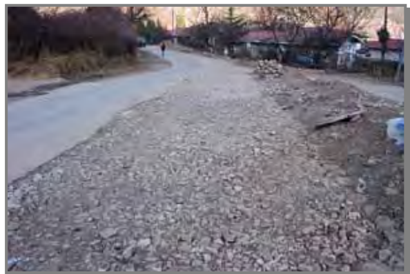
【Photo-22 :Road surface after removal of pitching】
