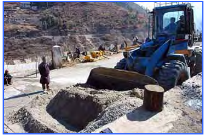
[Photo-15: Crosscut blending of subbase material]
