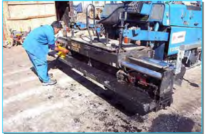
[Photo-12: Cleaning of paving machinery]
