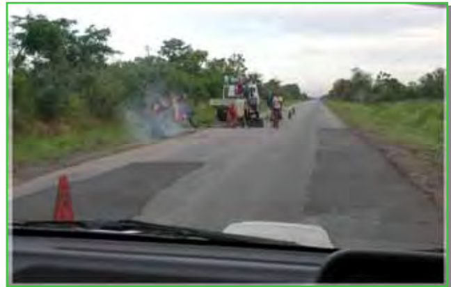
[Photo-46: Maintenance of East Africa transcontinental Express highway]
