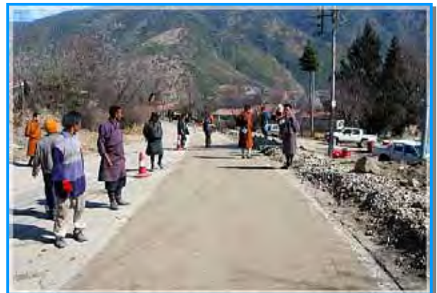
[Photo-29: Paved road after compaction]
