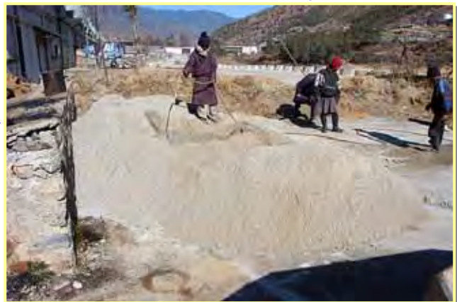
[Photo-14: Water content adjustment for shaping material]
