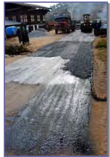
【Photo-42: Overlay pavement site in Hesothangkha 50 maintenance staff are working】
