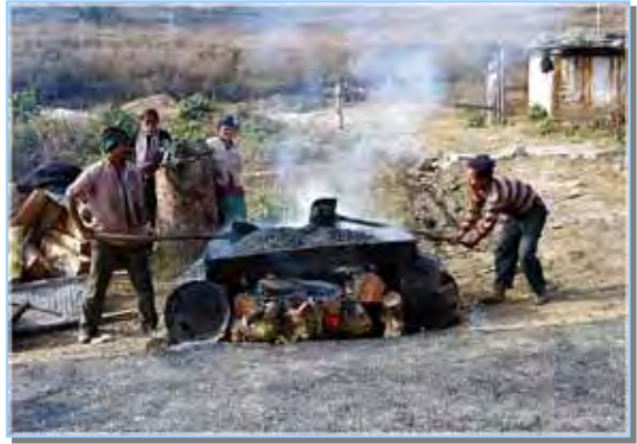
【Photo-40: Hot mixing on site】
