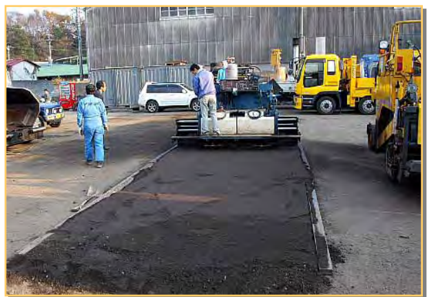
【Photo-8: Field exercise of finisher operation in Japan】
