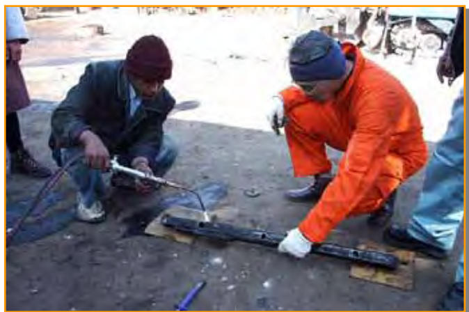
[Photo-11: Repairing side cover]
