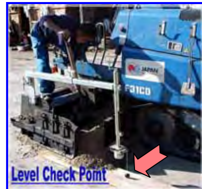
[Photo-16: Level check mark]
